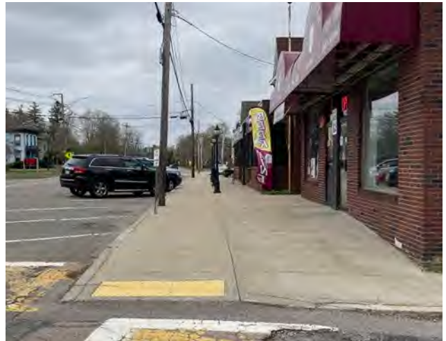
Concrete sidewalks are generally in good condition in the study area
