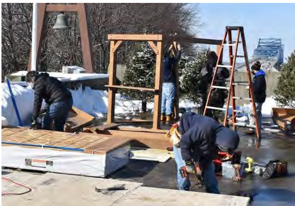
Volunteers helped build the “set” for the weekend activities.
