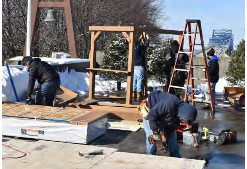
Volunteers helped build the “set” for the weekend activities.
